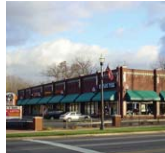
Bringing a portion of the building close to the street is encouraged whenever possible. Awnings providing visual interest
