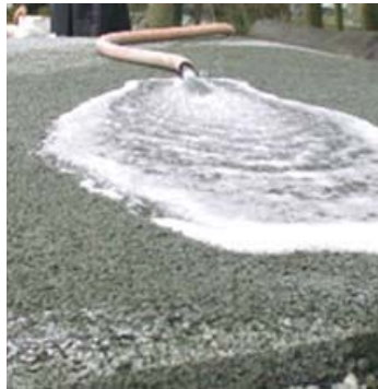
Permeable asphalt, provides an alternative to traditional, less permeable asphalt. On-site stormwater management methods should be used to protect local waterways
