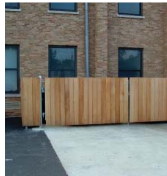
Service features such as garbage containers should be shielded from view in an enclosure compatible with the building architecture
