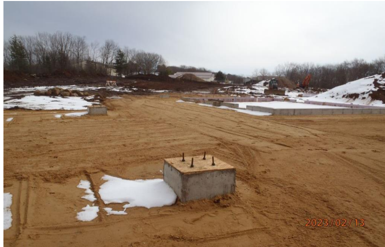
Building backfill around shelter.
