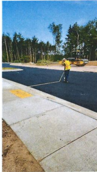
Parking lot paving.
