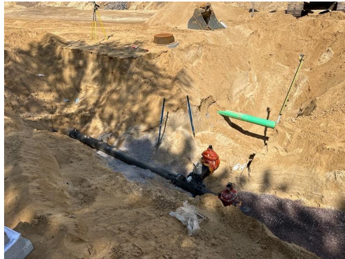
Water Main Installation at Prairie Hill Village Development August 2024
